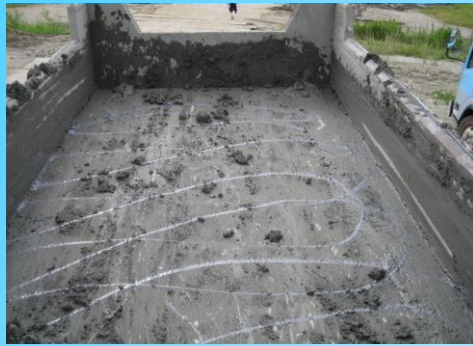
Apply an appropriate amount of Mud Suberu L on bed of dump
