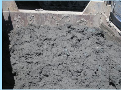
Loading of soil
